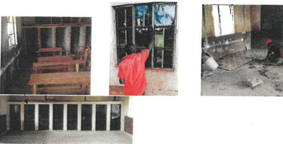
Power points installed
